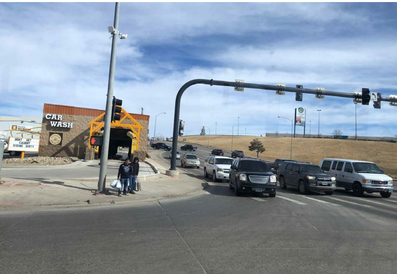
Some larger intersections, such as E. Second St and Wyoming Blvd shown here, have long crossing distances with a lack of pedestrian safety counter measures such as curb extensions, high visibility crosswalks, and refuge islands.
